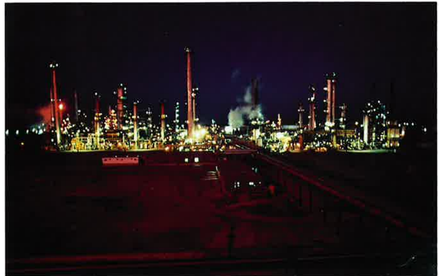
Bright, low-cost lighting is achieved with mercury-vapor lamps.
